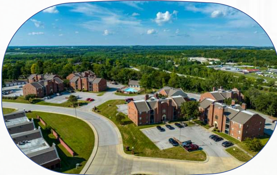
Oaks at Platte City 212 Units $19.2M
